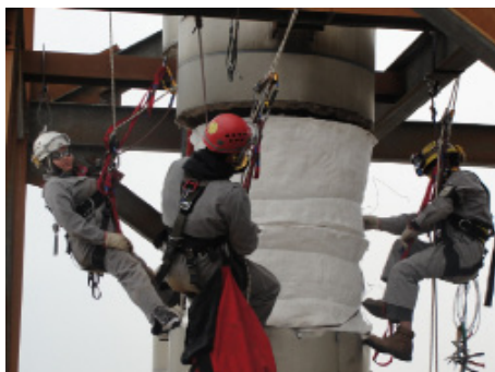
Figure 3: Insulation removal and repair
